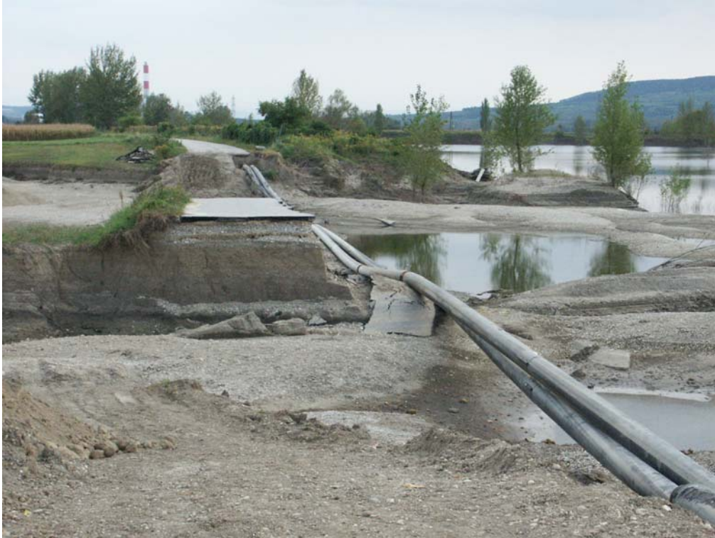
Figure 1: Broken road embankment and pipes for district heating, near Stratzdorf
